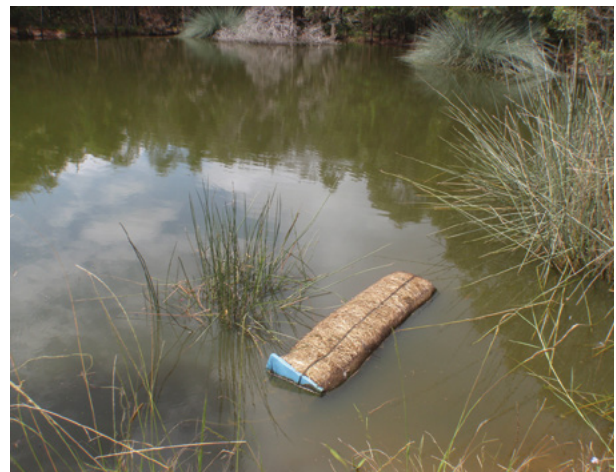
Figure 5.29 Installation of barley straw
