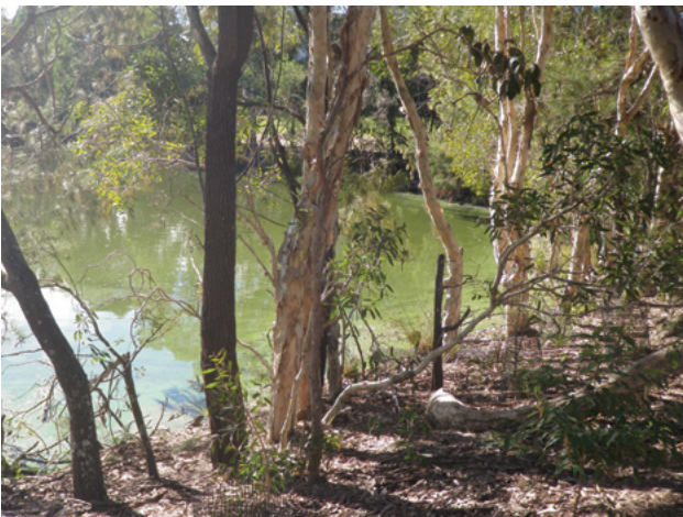
Figure 2.2 Farm dam in poor condition
