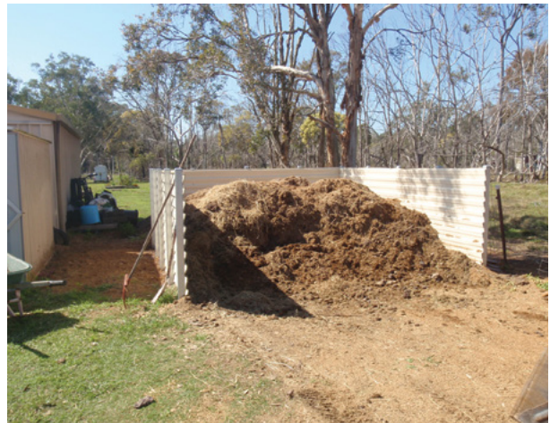
Figure 5.23 After - a manure compound for storing and composting manure
