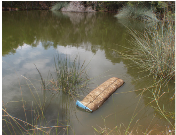
Figure 5.29 Installation of barley straw
