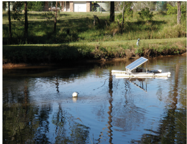
Figure 5.39 Solar water circulation system
