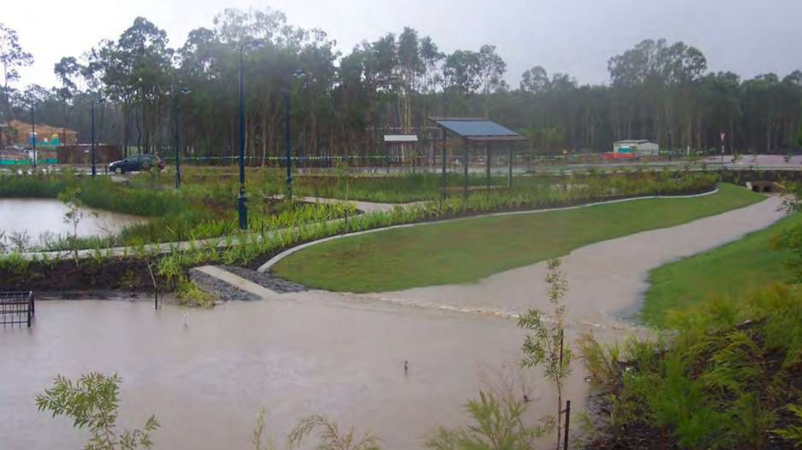
FIGURE 20 Photo spillway weir outlet
