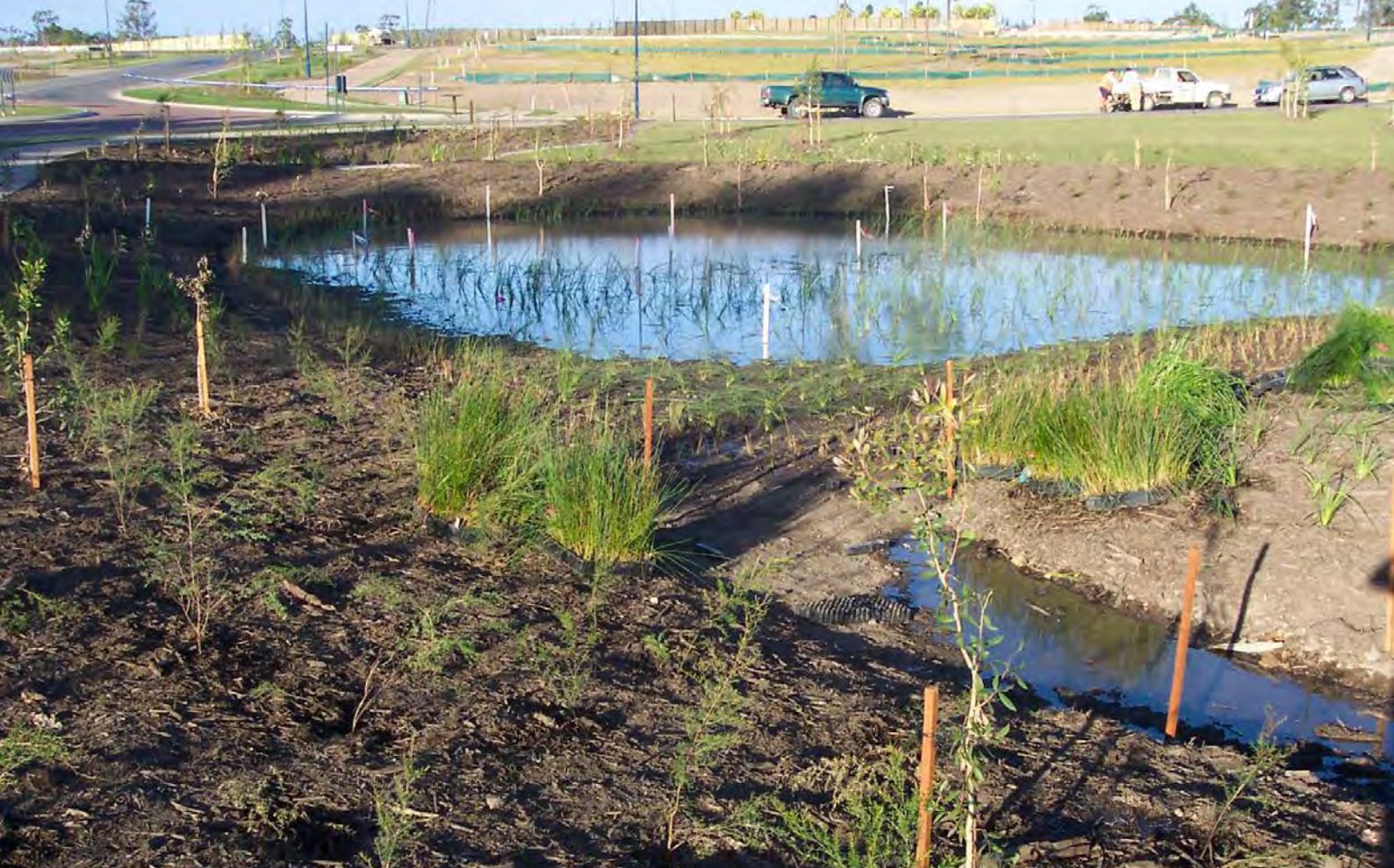
Figure 45 Plant setout and planting
