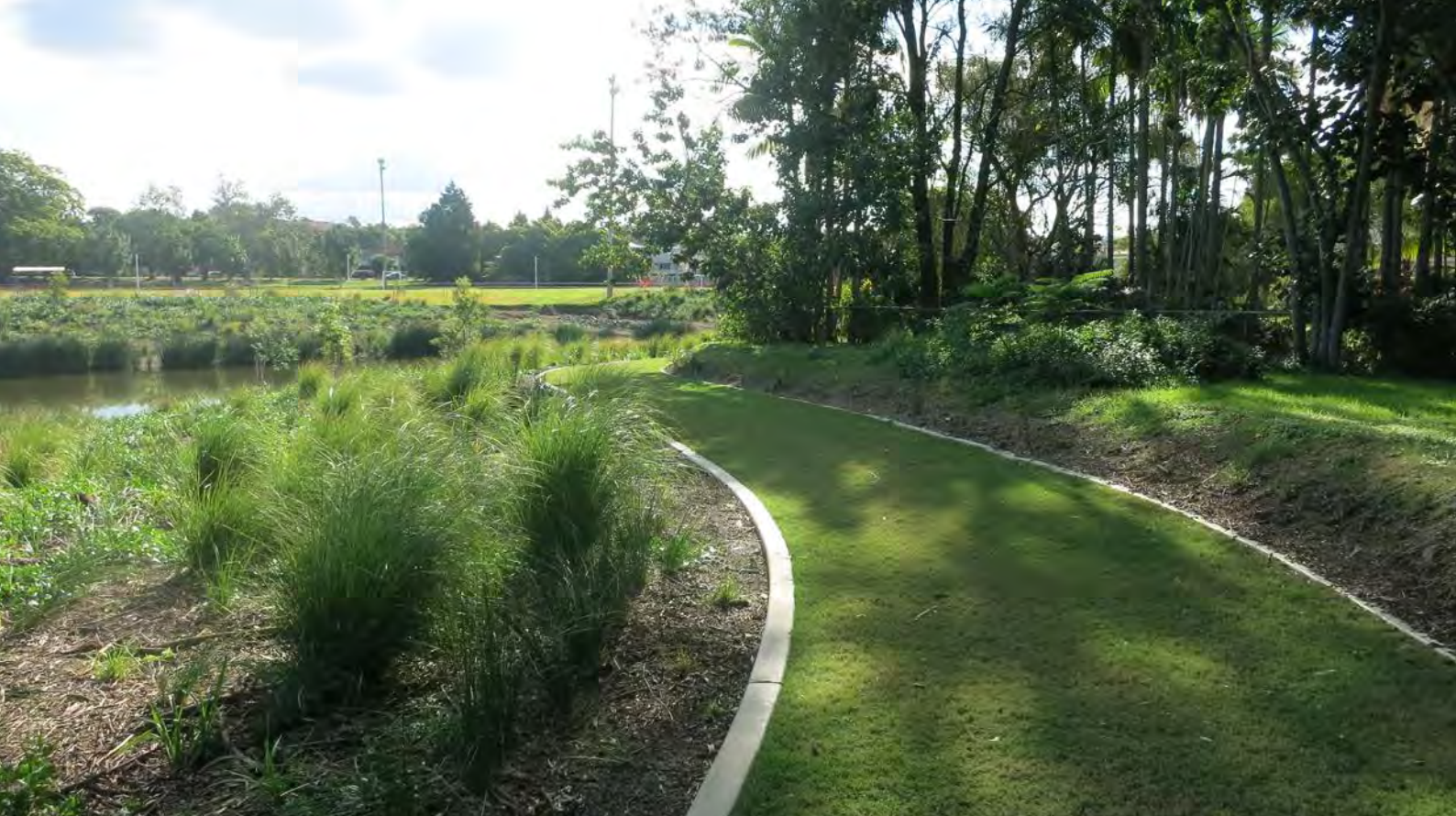
FIGURE 37 Maintenance Track – Reinforced turf
