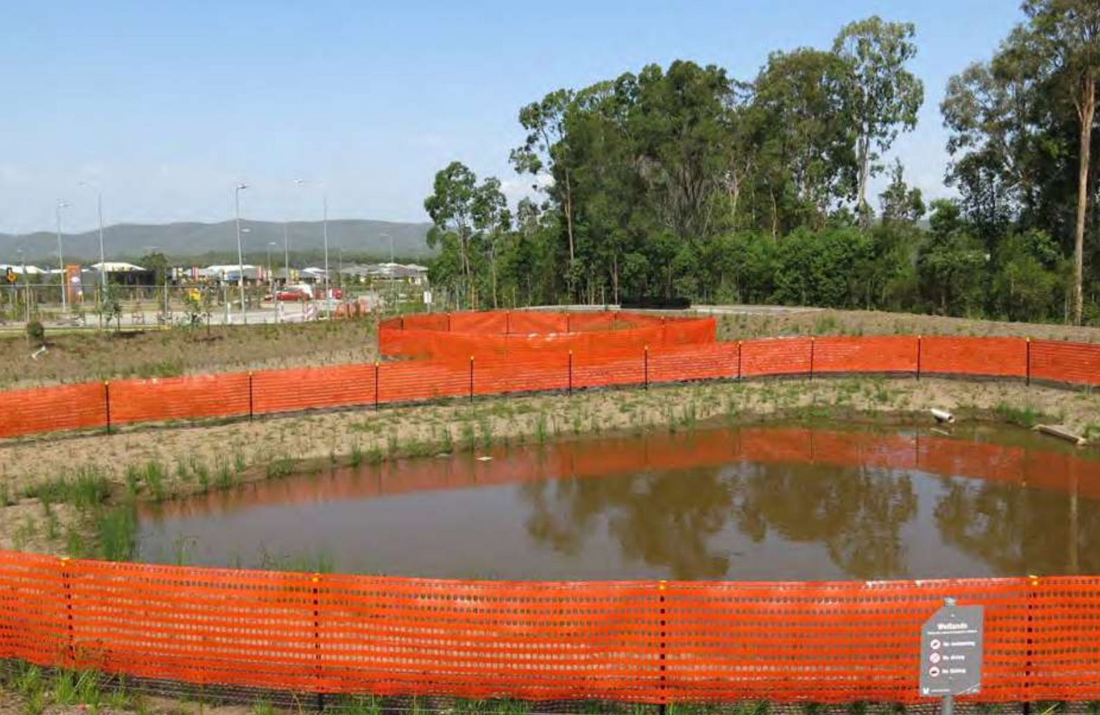
Figure 3 Example of temporary fencing during plant establishment
