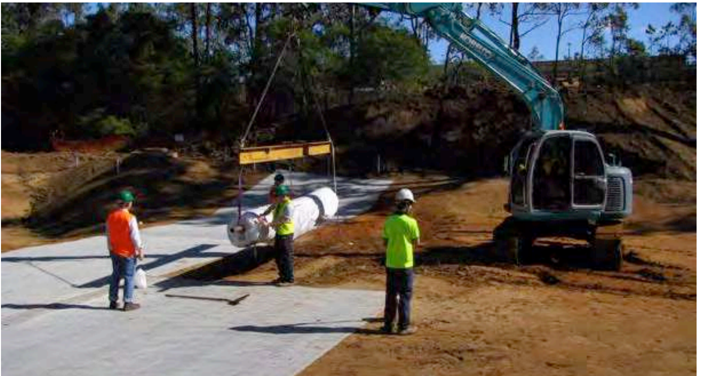
FIGURE 40 Synthetic liner installation
