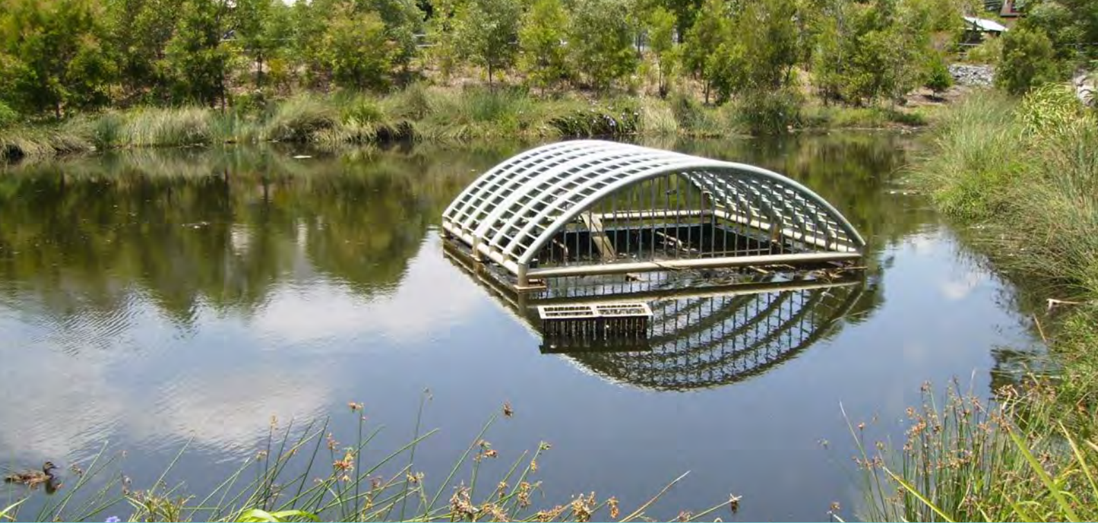
FIGURE 18 Sediment basin overflow pit
