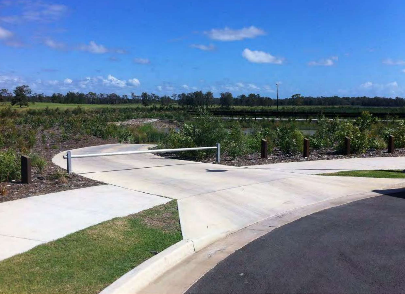
FIGURE 35 Site access and ramp to sediment basin
