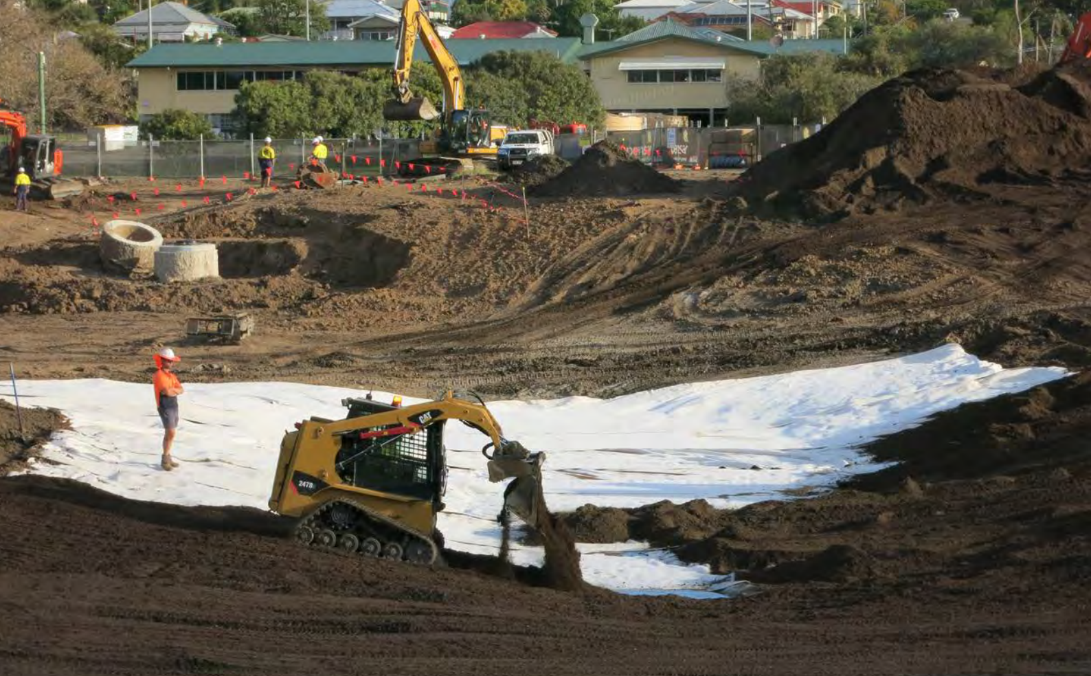
FIGURE 41 Topsoil installation
