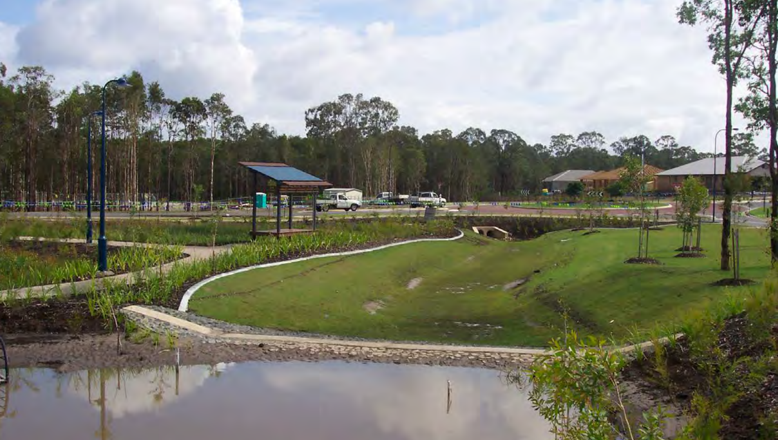
FIGURE 21 Constructed Wetland Bypass Weir and Channel Configurations
