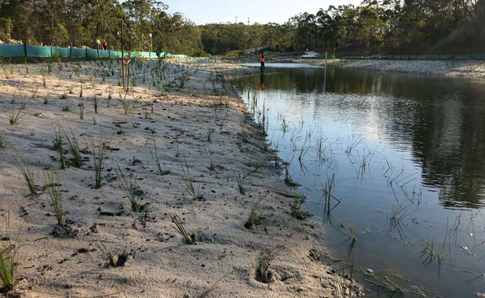
FIGURE 27 Safety Bench during plant installation
