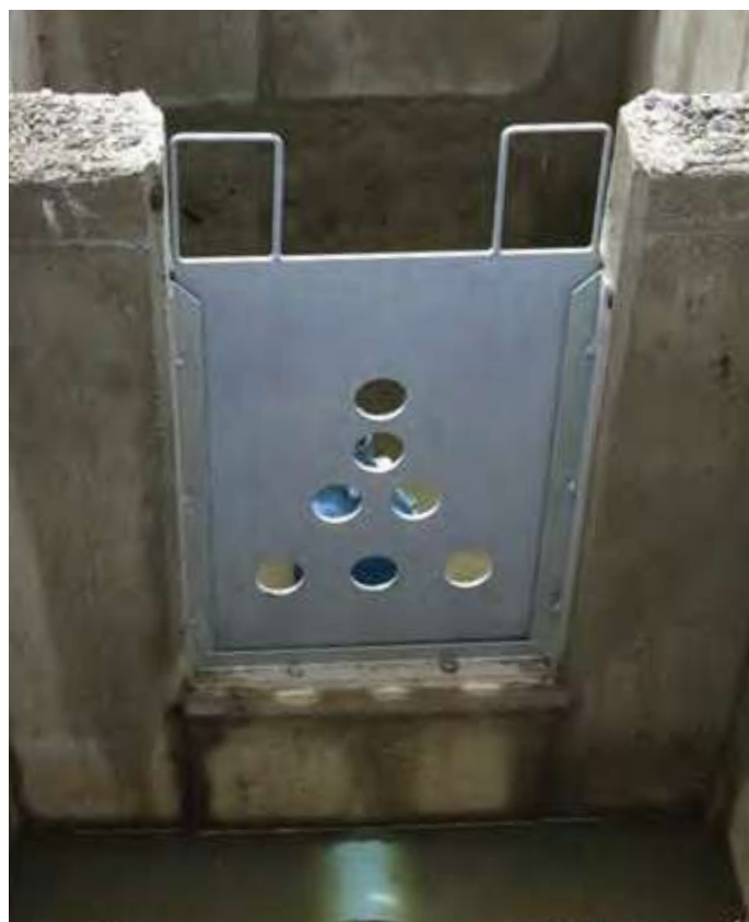
FIGURE 32 Plate riser Photo: Jason Sonneman - DesignFlow
