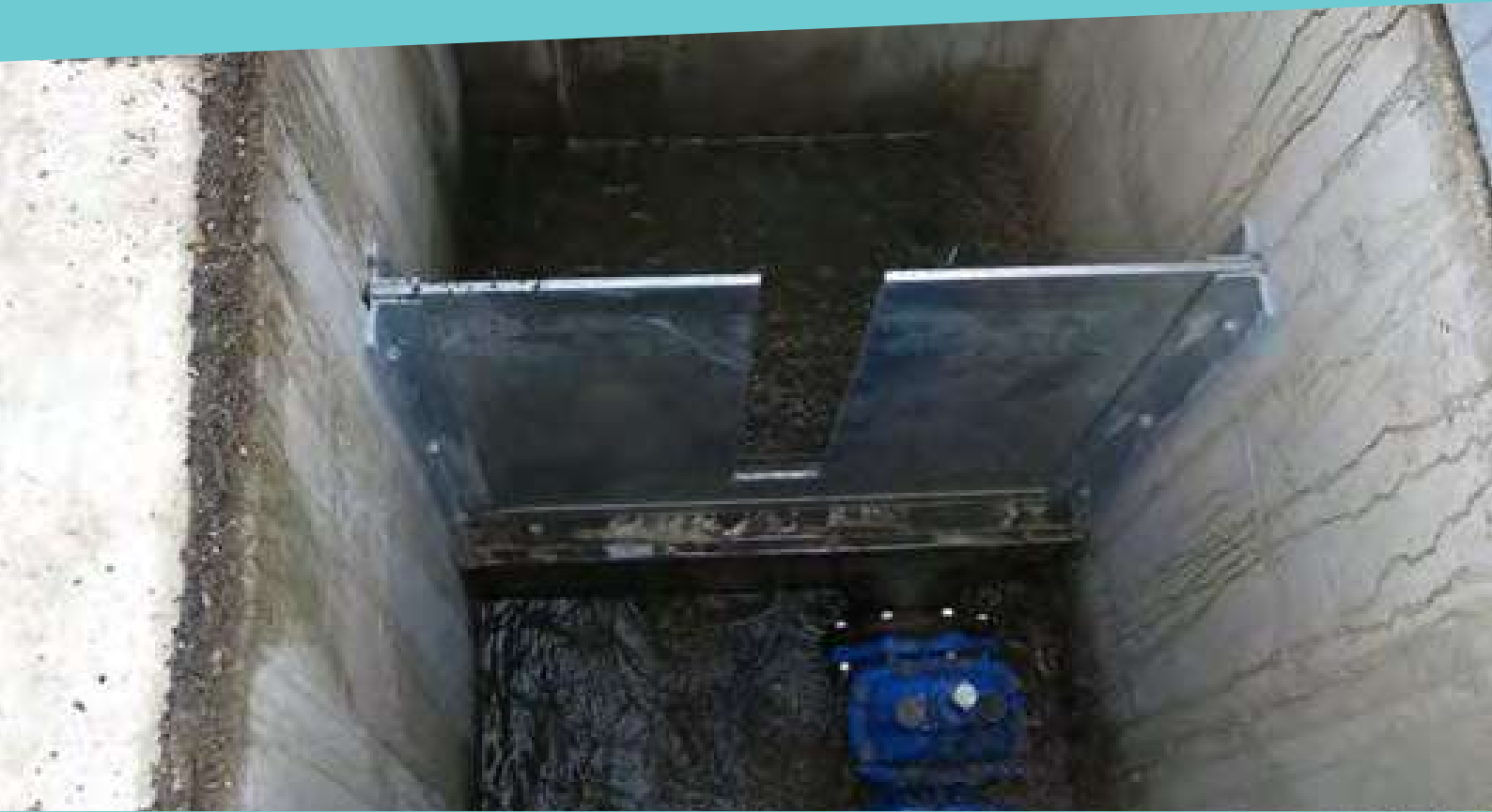
FIGURE 33 Slot weir outlet
