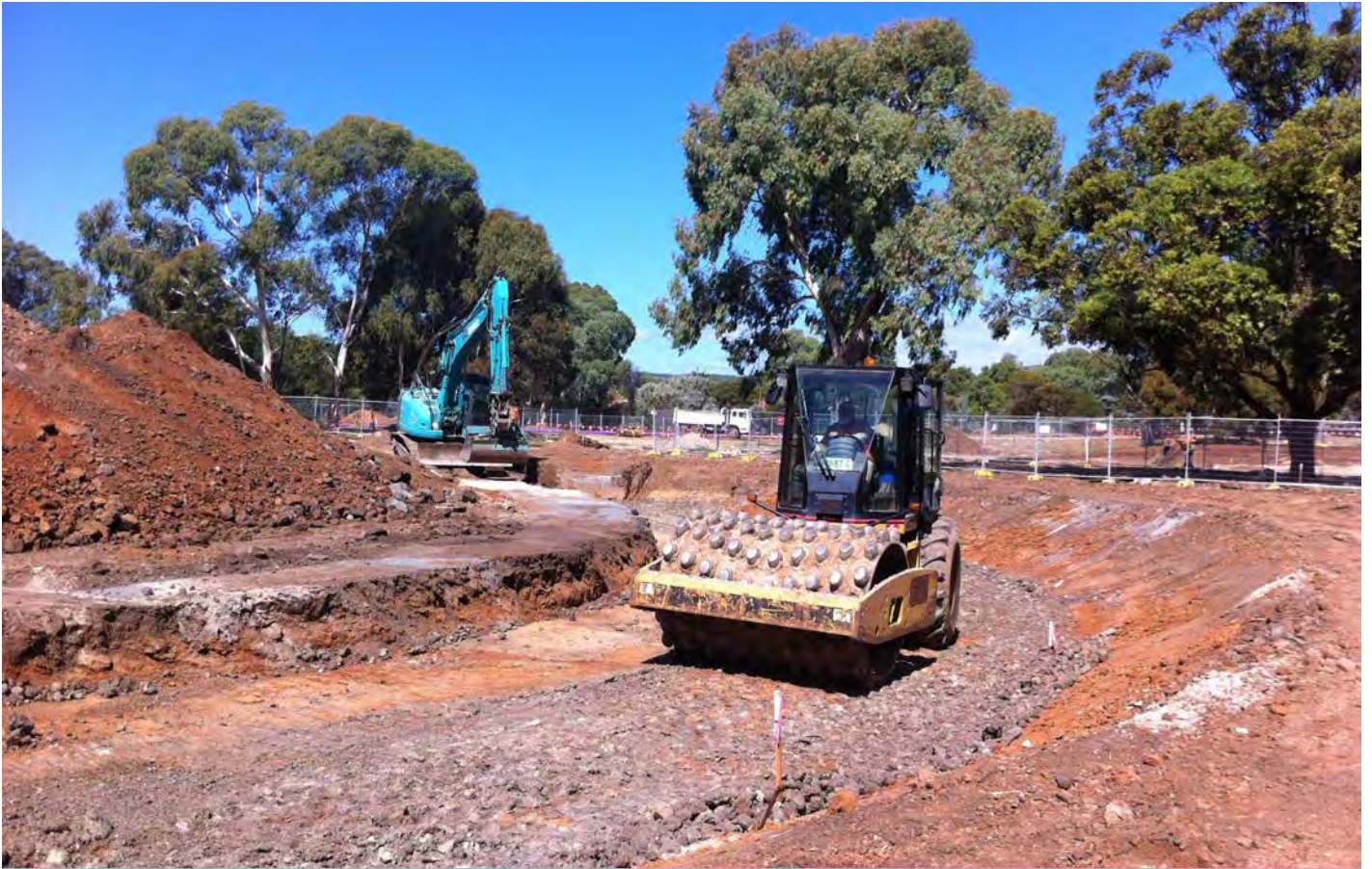
FIGURE 39 Clay impermeable liner installation
