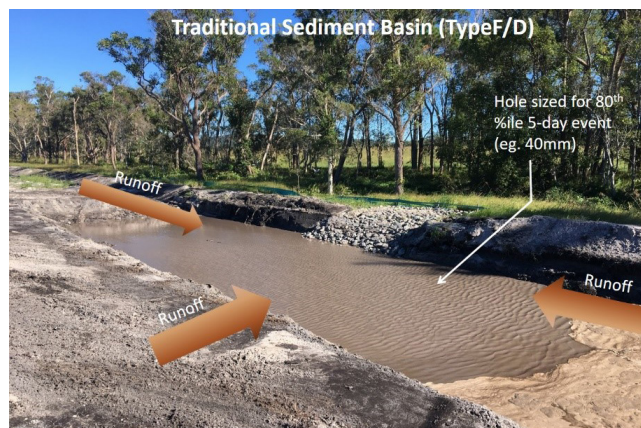
Figure 1 – Steps in Traditional batch sediment basin operation
