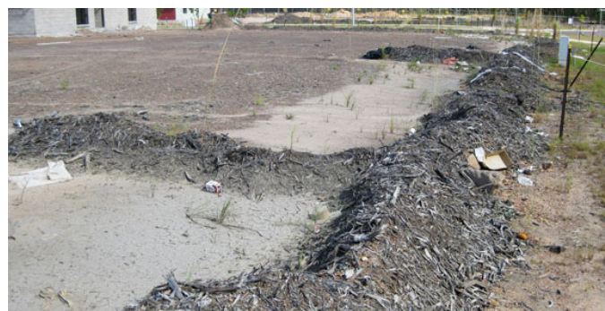
Mulch berm with upslope 'return' being used on small, flat house lots. (Source: Catchments and Creeks Pty Ltd)
