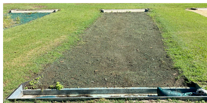
Spray on soil binder (polymer) (Source: Healthy Land and Water)
