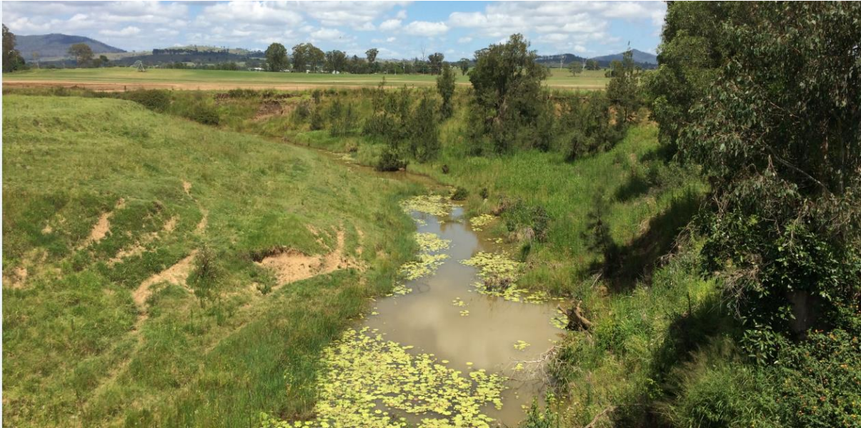
Figure 50. Allan Creek – classified as slightly confined – floodplain/terrace with moderate instabilities of inset units. Field verification indicated bank instabilities along the lower bank which comprised of inset benches and no observed lateral adjustment of macrochannel bank.
