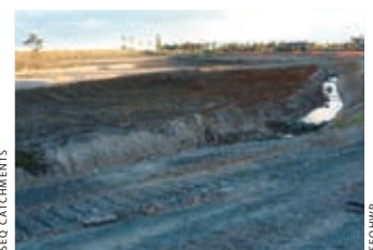
Construction without Water Sensitive Urban Design allows diffuse pollution to enter waterways.
