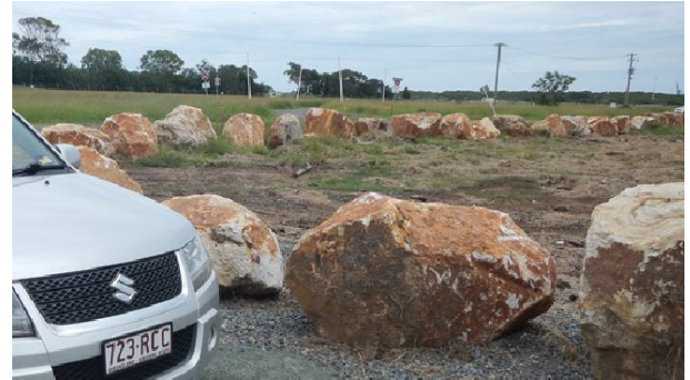
Large rocks were used to demarcate the intertidal zone and prevent vehicle access to give the mangroves and saltmarsh a chance to recover.
