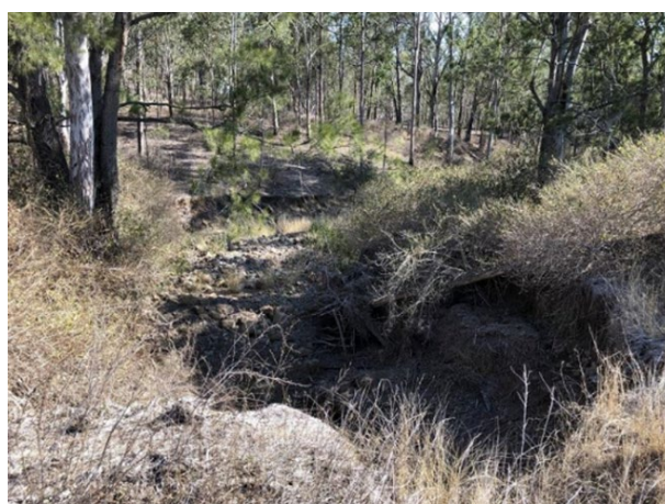
Figure 1. The erosion site before restoration works.
