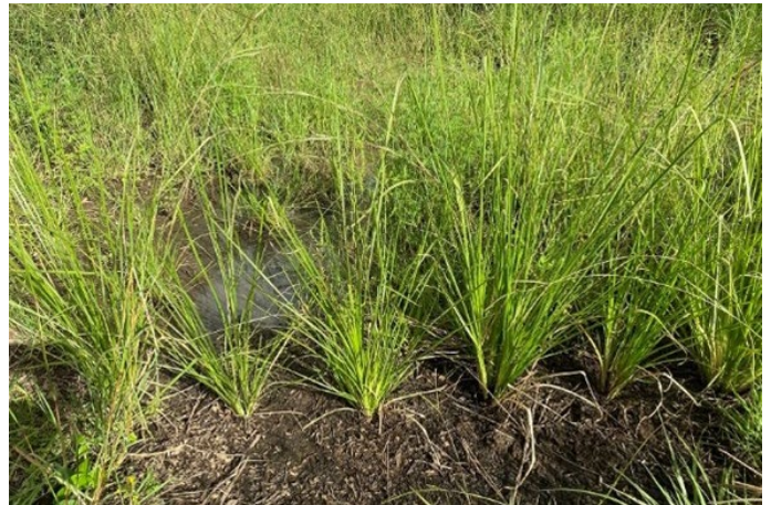
Figure 7. Vetiver hedges were installed to slow and redirect the flow of runoff entering the chute.
