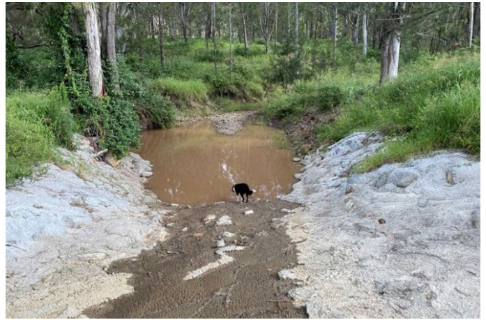
Figure 9. Concrete was used to secure the rock and stabilise the chute.
