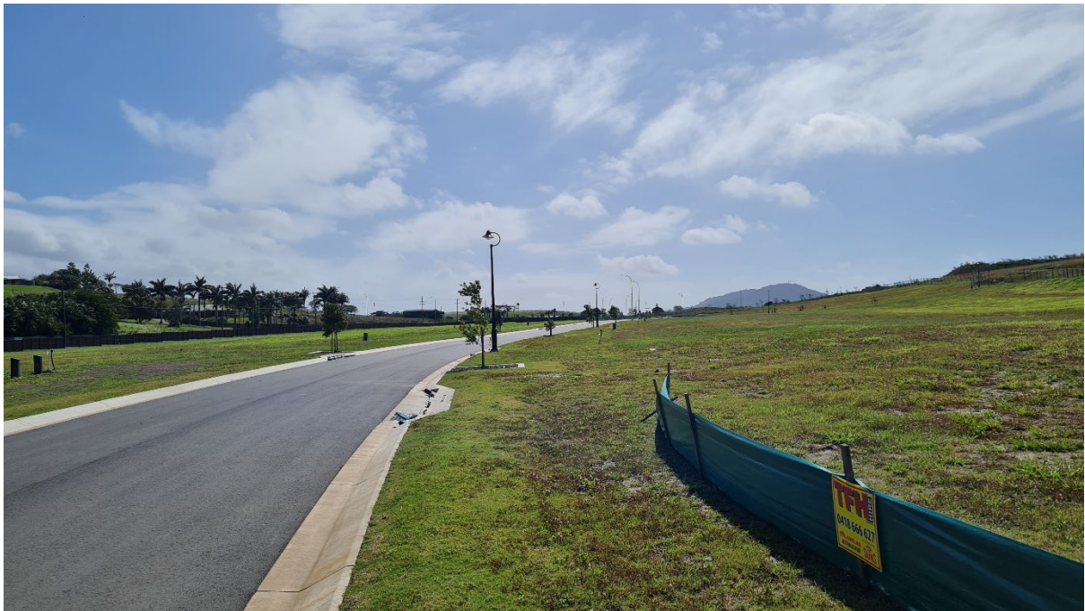
Stabilised finished lots
